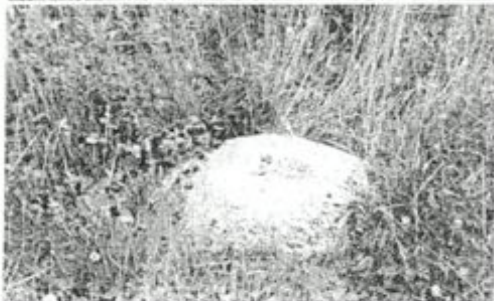
Top - Photo 1. Dunrobin site. A typical concrete monument with the steel cut down to the concrete. (Photo taken 24 July 95).
